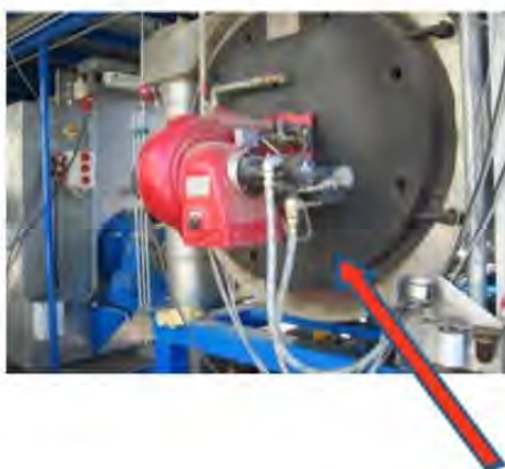
The Fuel Burner at the TDU heater
