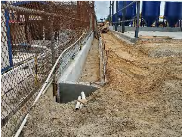
Figure 4-2: Main Internal Drain under Construction
