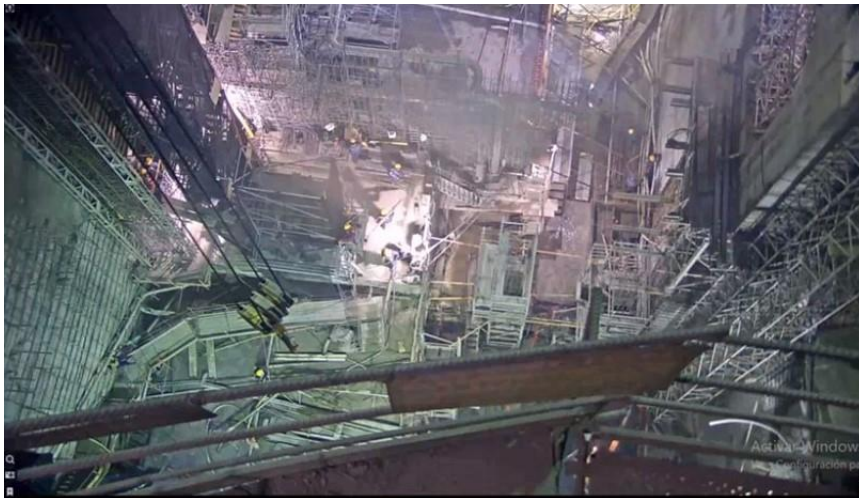
Figure 46: Civil works on the area of Control Room North
