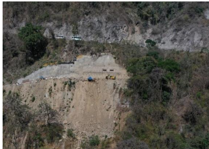
Figure 37: Ongoing slope reinforcement works
