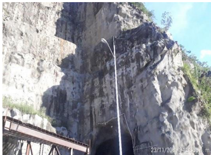
Fig. 53: Intake gates: Installation of final lighting in the external area
