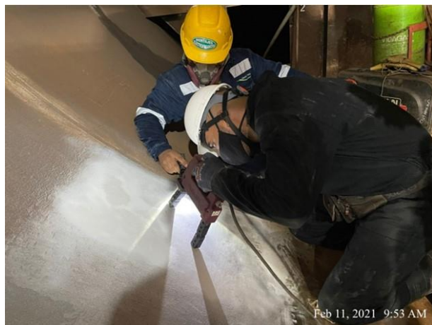
Figure 55: Lower elbow: steel lining testing
