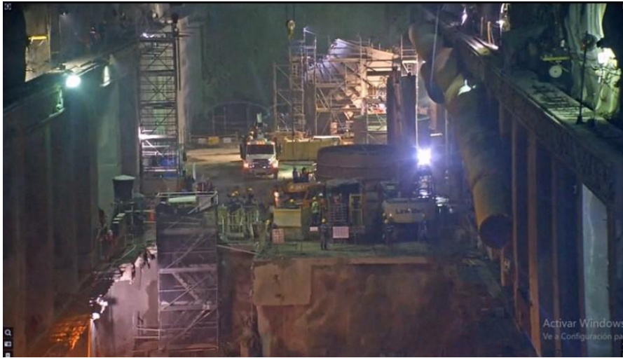
Figure 45: Loading bay and unit 5 and 6 bays utilised as additional loading bays
