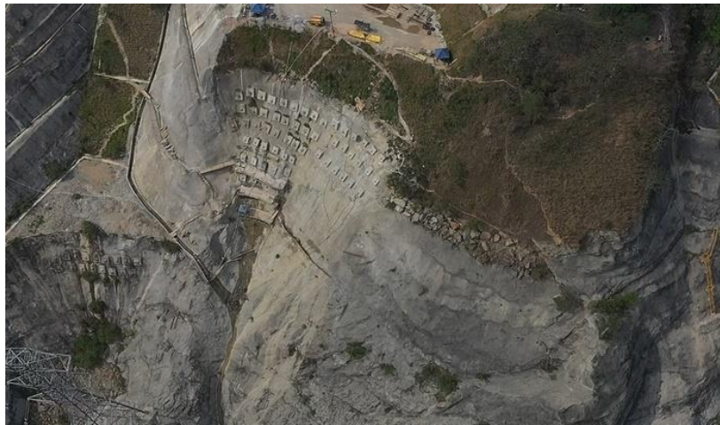
Figure 52: The stabilization works [switchyard on the bottom left corner – archive]
