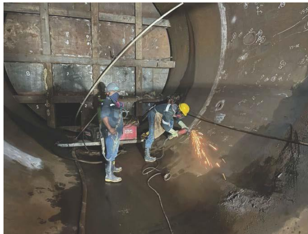
Figure 54: Lower elbow: steel lining repairing
