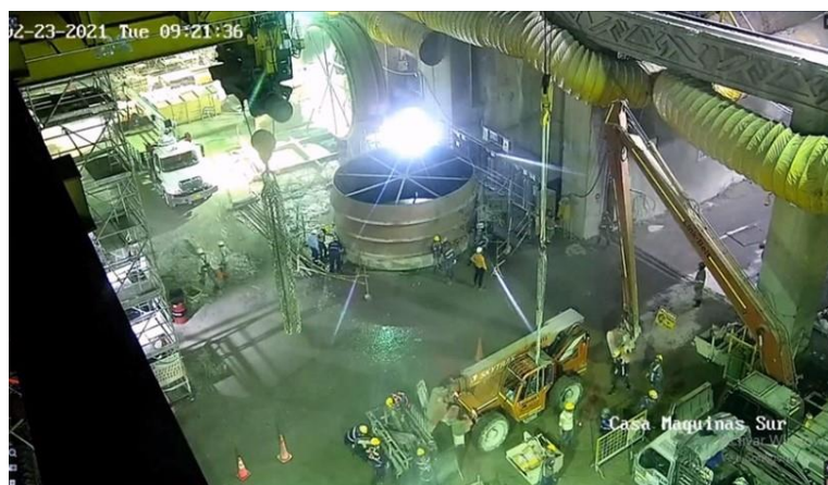
Figure 44: Loading bay and access tunnel seen from South Powerhouse
