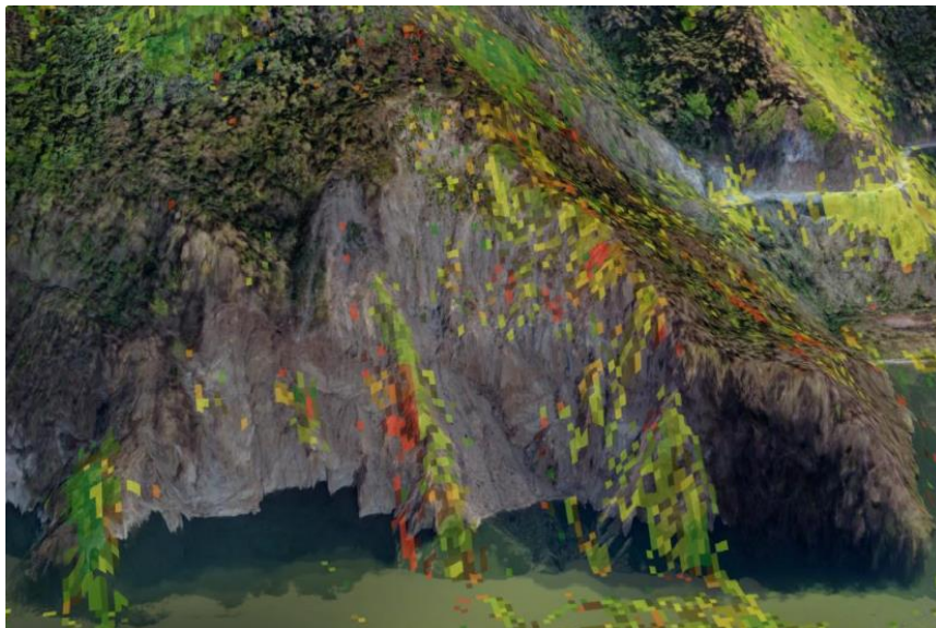
Figure 35: The upstream right-side slope. Satellite monitoring. Red points correspond to displacements.
