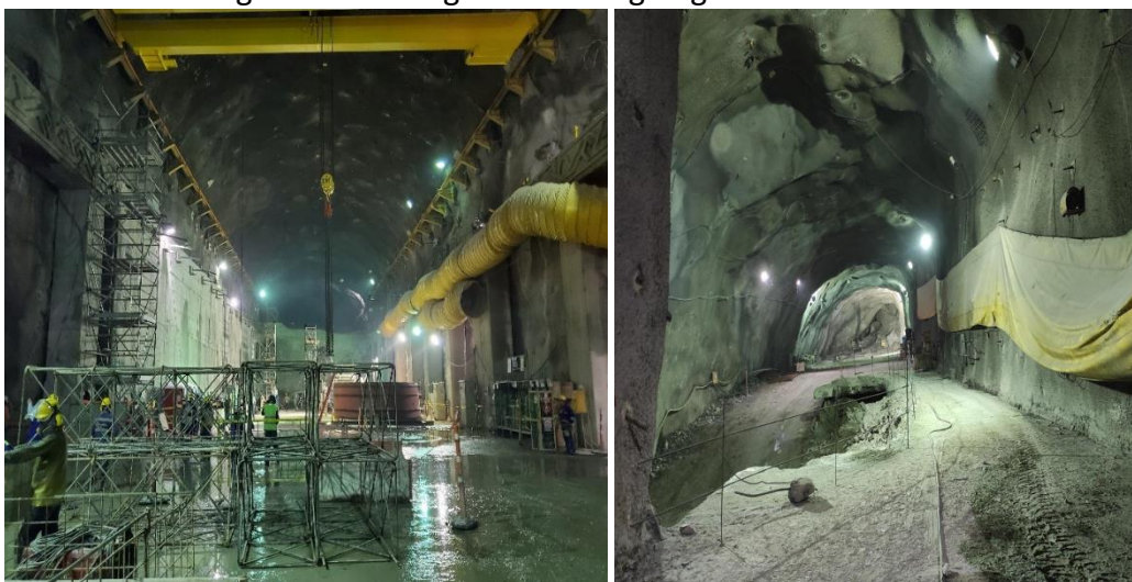
Figure 17: Machine Hall, generator level (left) and backfilled North Surge Shaft (right)
