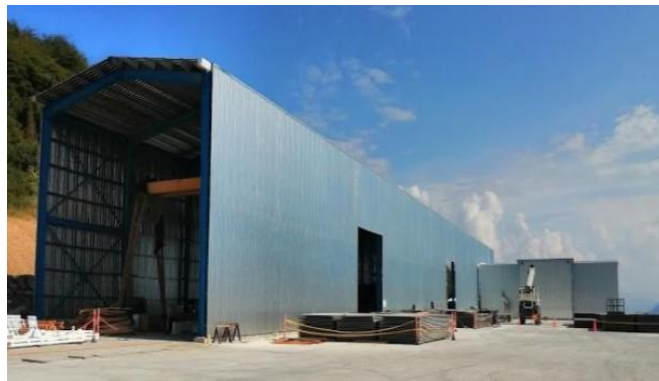
Figure 57: ATB workshop completed
