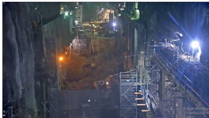
Figure 43: Unit 3 and 4 demolition of concretes
