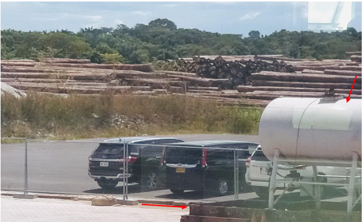
The log yard and the storage tank for diesel with containment bin (see red arrow).
