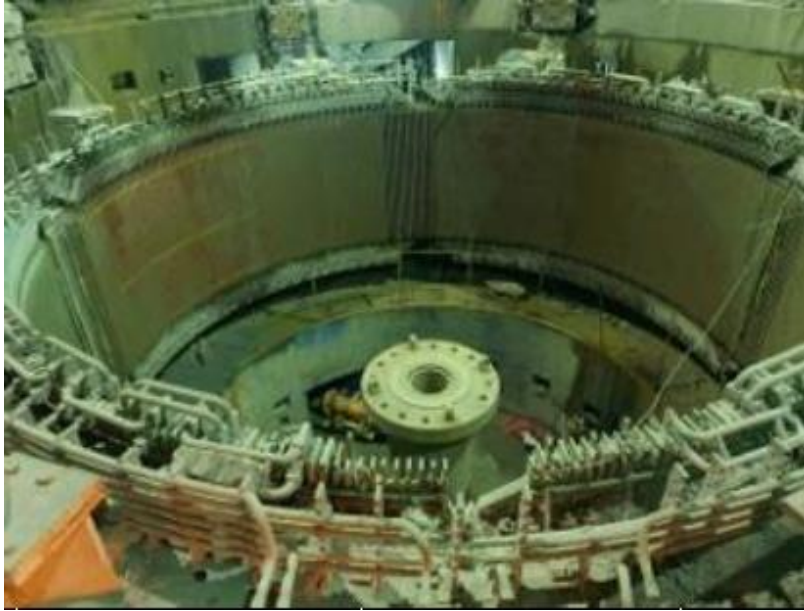
Figure 17 – Stator of Unit 3 clean and ready to be removed.
