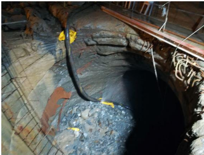
Figure 13 – Remaining of Unit 4 draft tube.
