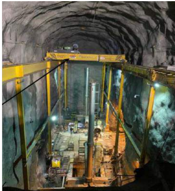
Figure 31: Removal of the crane from the GAD control chamber
