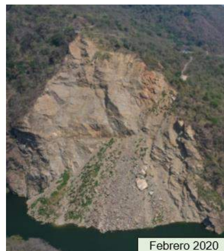
Figure 20: Instabilities near the complex of the project, at the left side, over of the reservoir, Left, at 0+900 to 1+290 and right at 2+255
