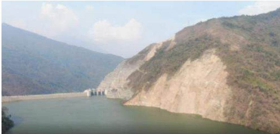
Figure 19: The destabilized area above the two diversion tunnels. In the far upper end the slopes of Romero, before the reshaping and treatment
