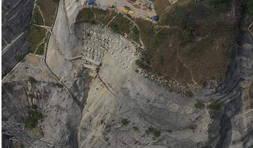
Figure 27: The stabilization works [switchyard on the bottom left corner]
