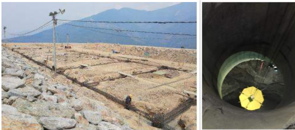
Figure 29 - Left: penstocks assembling area. Right: shafts 1 and 2, steel lining installation
