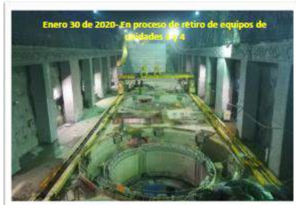
Figure 24: Removing Unit 3 and 4 equipment as scrap material
