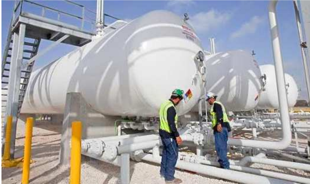
Figure 31: Physical inspection of LPG Tanks and Aboveground Piping
