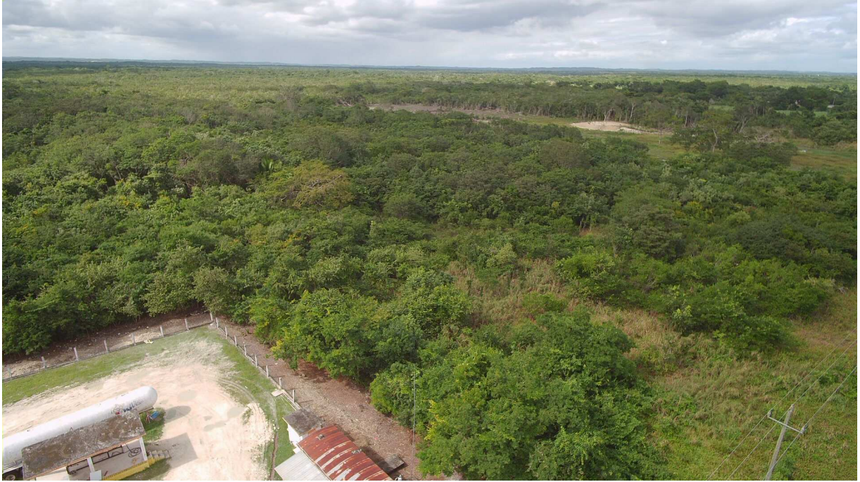
Photograph 27B – Orange Walk LPG Depot Site
