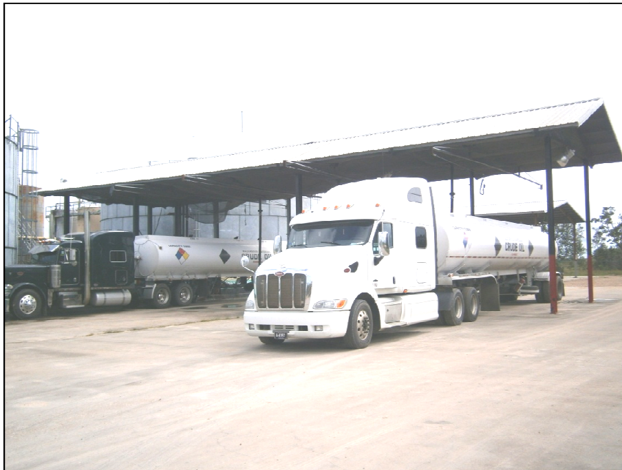
Photo 20 – Example of a Multi-Lanes Tanker Truck Loading Facility
