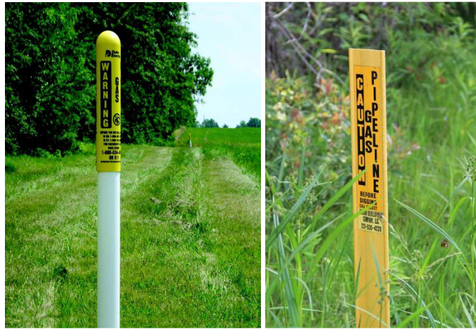
Photo #47: Examples of Gas Pipeline markers.
