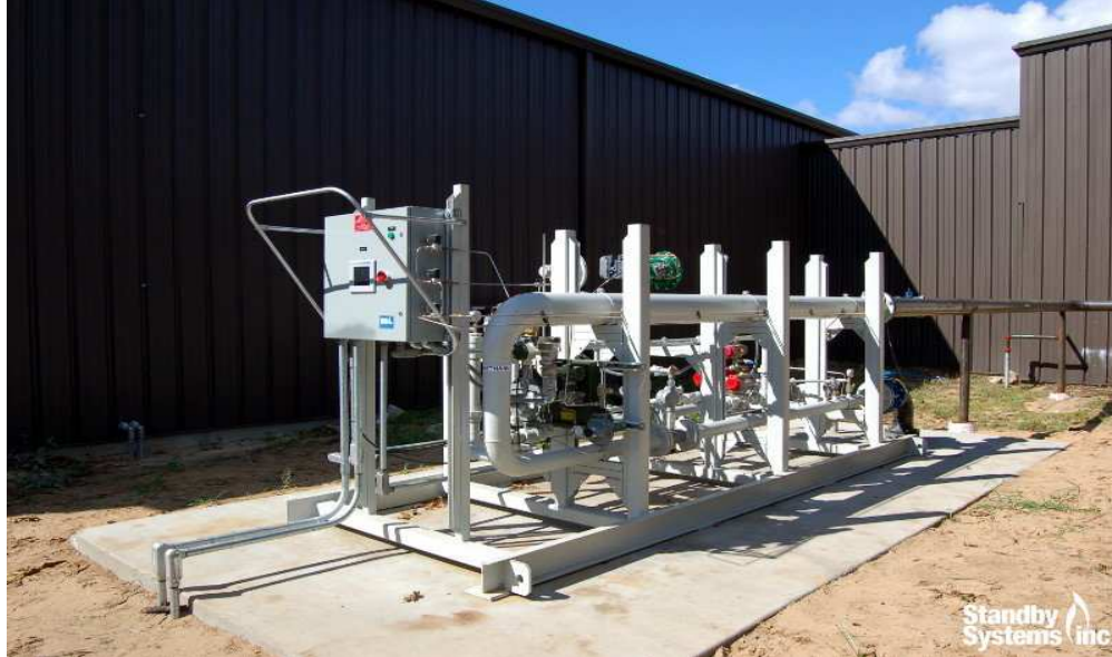
Photograph 13 – Example of Butane/Propane Blending Facility/Skid
