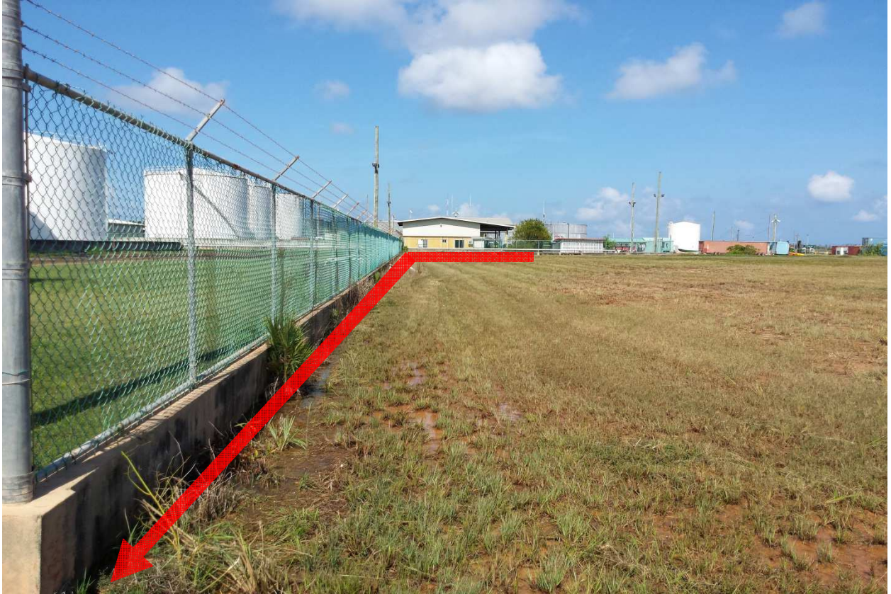
Photos #7: Proposed Pipeline route along outer perimeter of Petro Fuel Facility leading to BNGC tank farm
