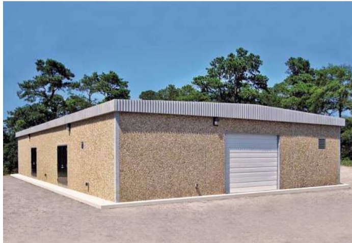
Photograph #12: Example of Ferro-concrete structure with cement roof
