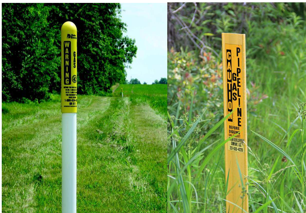
Photo #10: Examples of Gas Pipeline markers.
