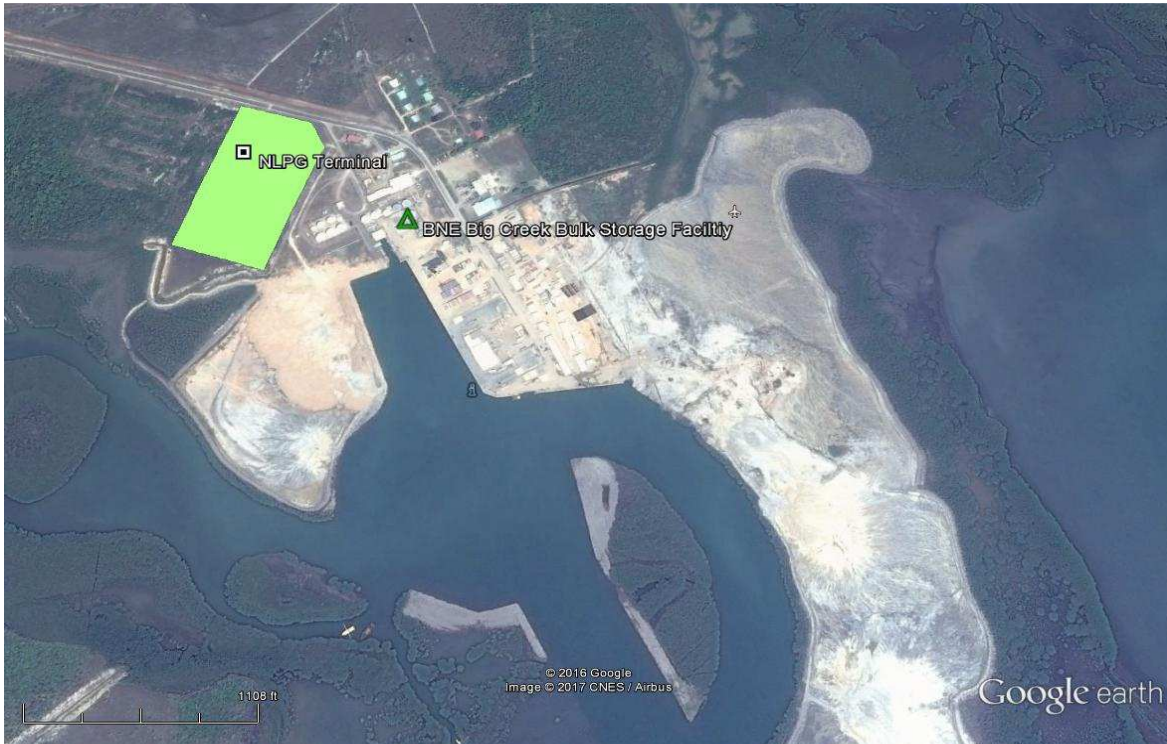
Fig. 5 - Proposed location of BNGC Terminal Storage Tank Farm (area highlighted in green)
