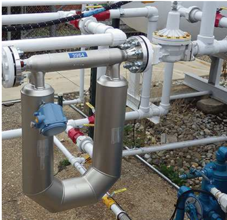
Photograph # 17: Example of a Coriolis Mass Flow Meter
