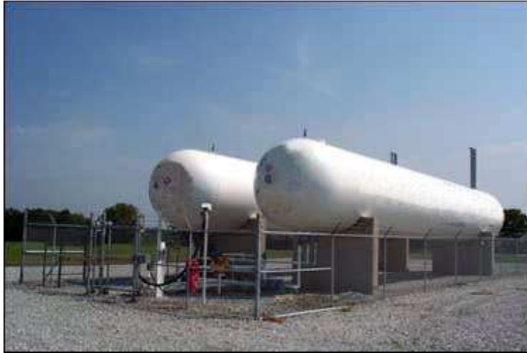
Photograph 20B – Security fence around LPG Tanks
