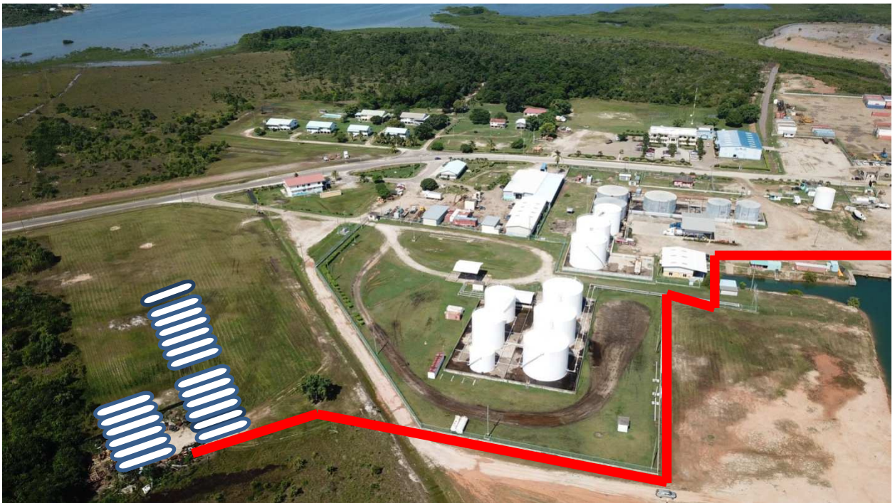
Photo #9: Pipeline route from berthing area to BNGC Storage Facility
