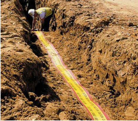
Photograph 45: Warning tape being installed one foot above underground pipeline
