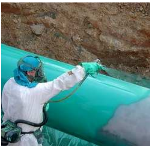
Photo# 41: Painting of Underground pipeline
