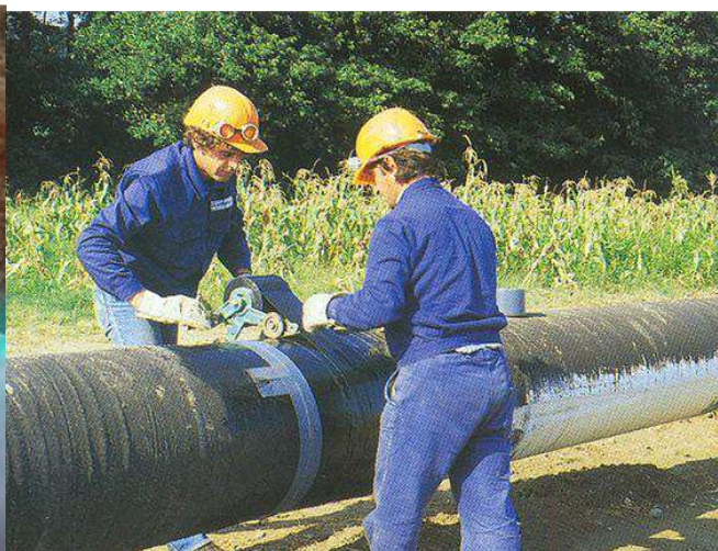
Photo#42: Wrapping Pipeline with Bitumen Tape
