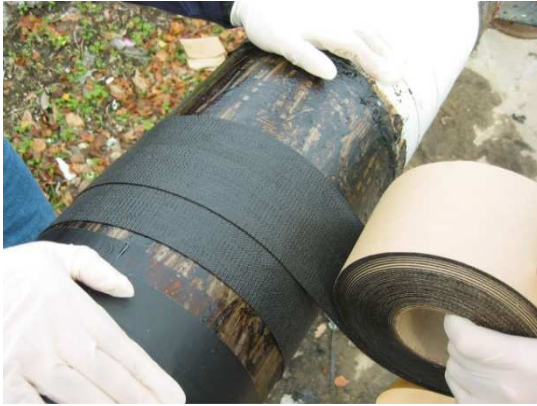
Photo # 43: Wrapping Pipeline with Grease cloth
