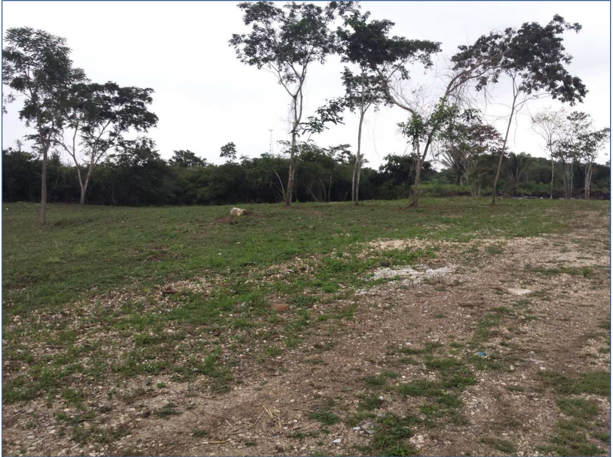
Photograph 27A: Cleared site for Central Region Depot
