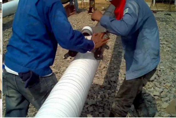
Photo #43A: Wrapping Pipeline with PVC-like Tape
