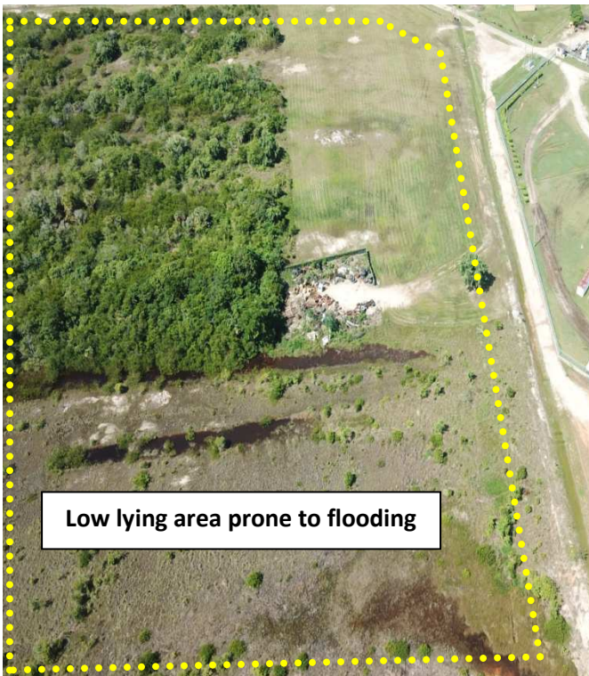
Photograph 29: Aerial view of Topography of BNGC Terminal Site.
