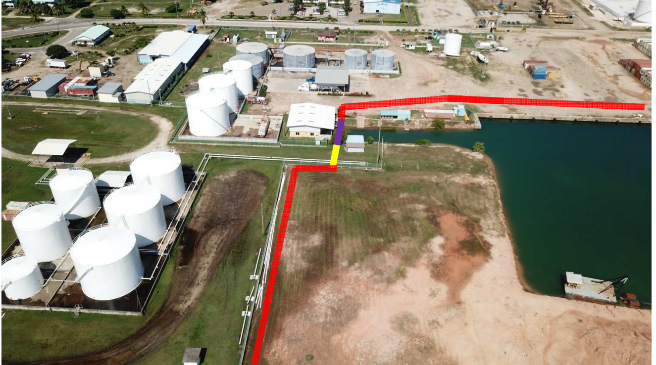
Photograph 5: Showing Pipeline Route from the Berthing facility over the water channel and through Petro-fuel facility.
