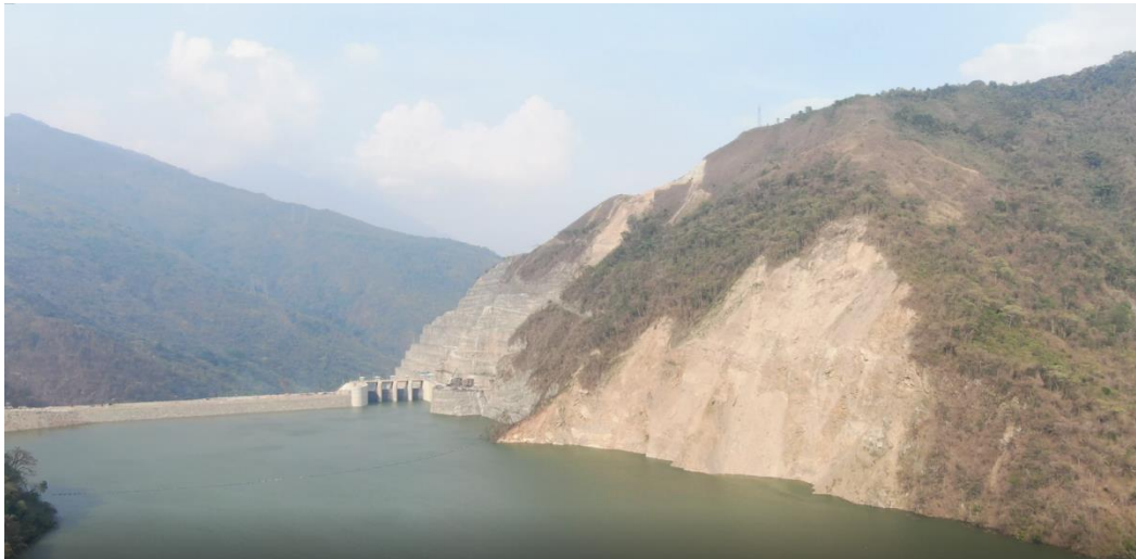
Figure No.14: The destabilized area above the two diversion tunnels. In the far upper end the shape of the “El Romerito” landslide
