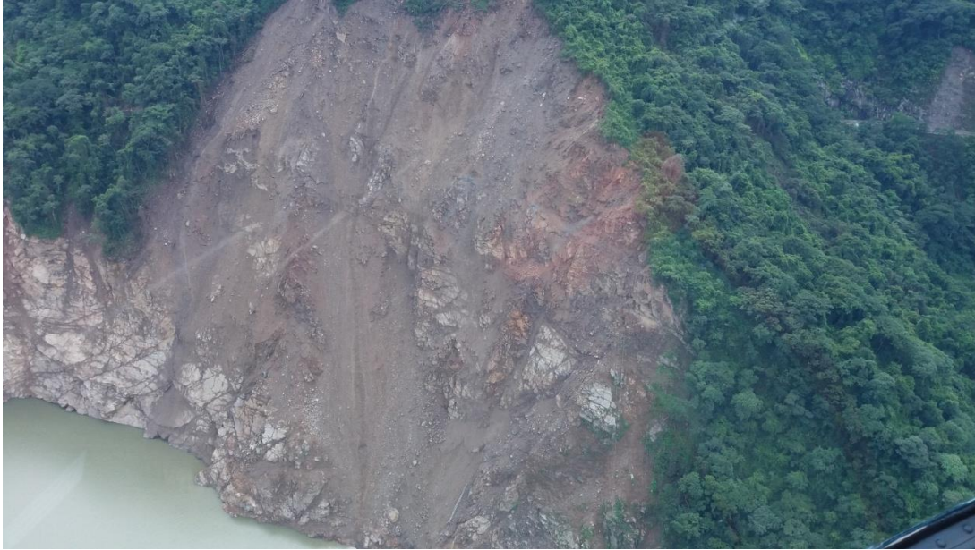
Figure No.7: Distressed rock mass and weathered zone. Landslide over the 2 diversion tunnels area. Photo on the 3rd August from the helicopter.
