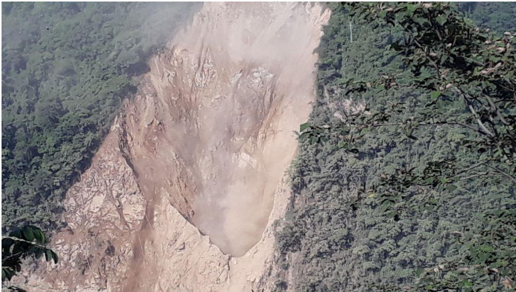
Picture No.2: Landslide and sinkhole at the diversion tunnel portals
