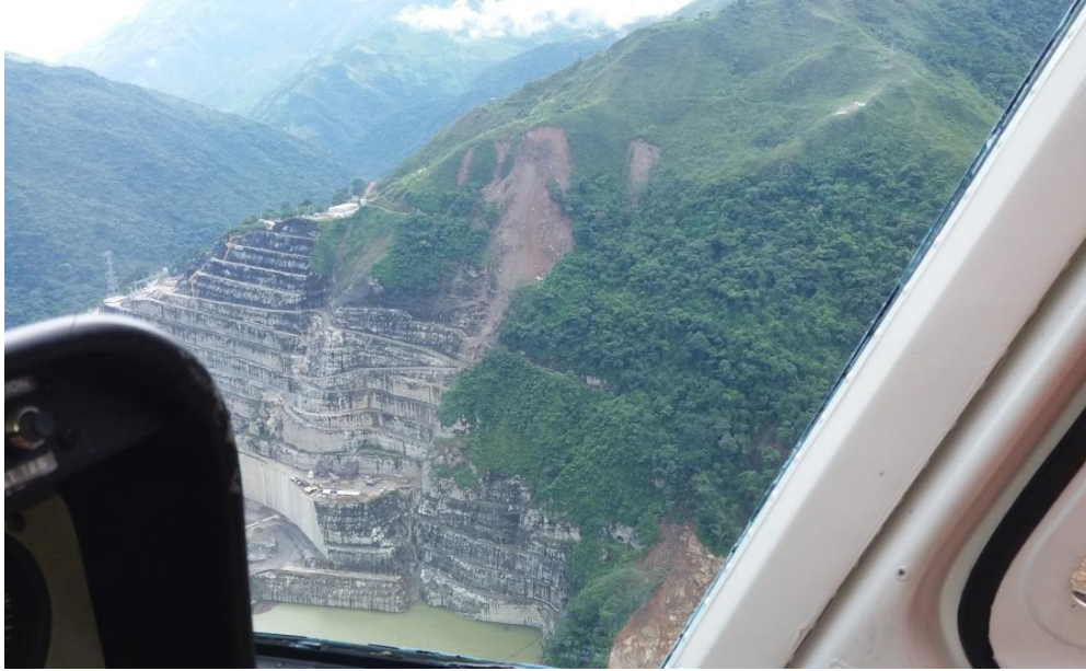
Figure No.13: The landslide over the intake structure is developed on the 26th of May. A concave form of the terrain uphill may denote the presence of an old slide (photo from helicopter August 3,2018)
