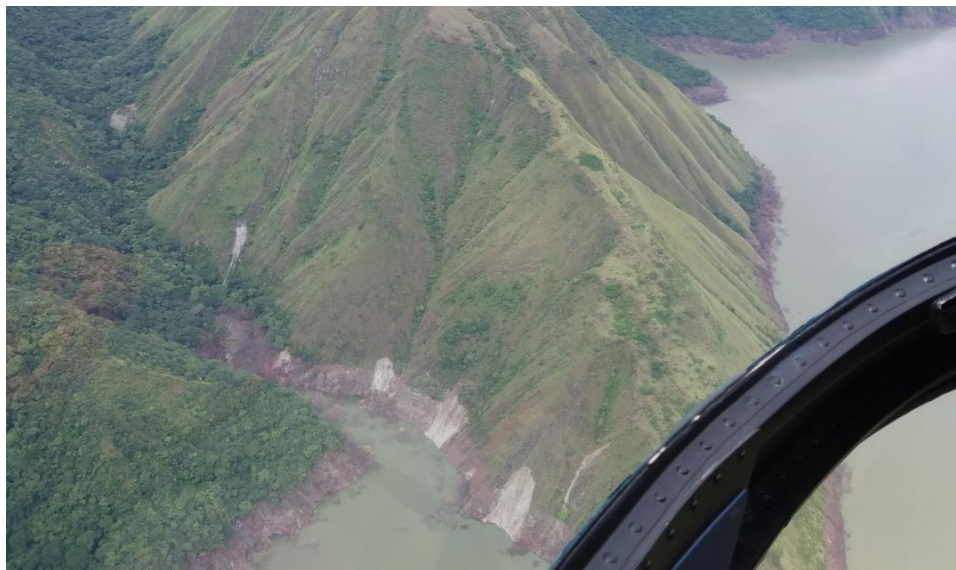
Figure No.19: Small landslides at the margin of the reservoir.
