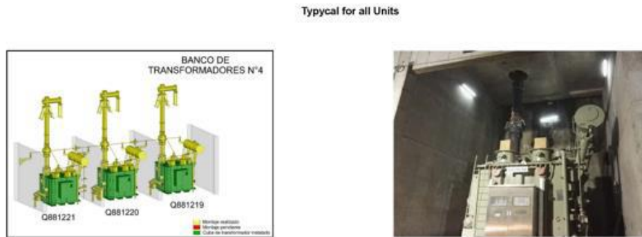
Figure No.24: Progress of installation of Transformers
