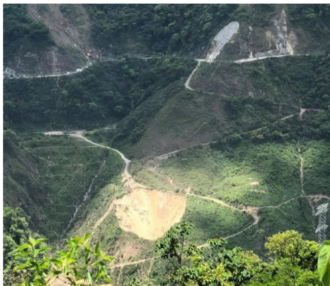
Picture No.1: Sinkhole above the ADT
