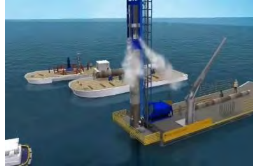
b. Pile driving
