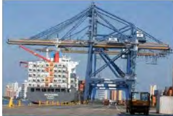
New Post Panamax Gantry Cranes
