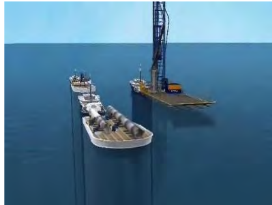
Figure Num. 3.23. Anchorage of barges and location and transport of piles
