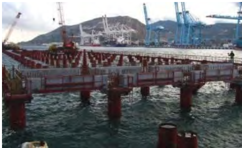
e. Installed beams
