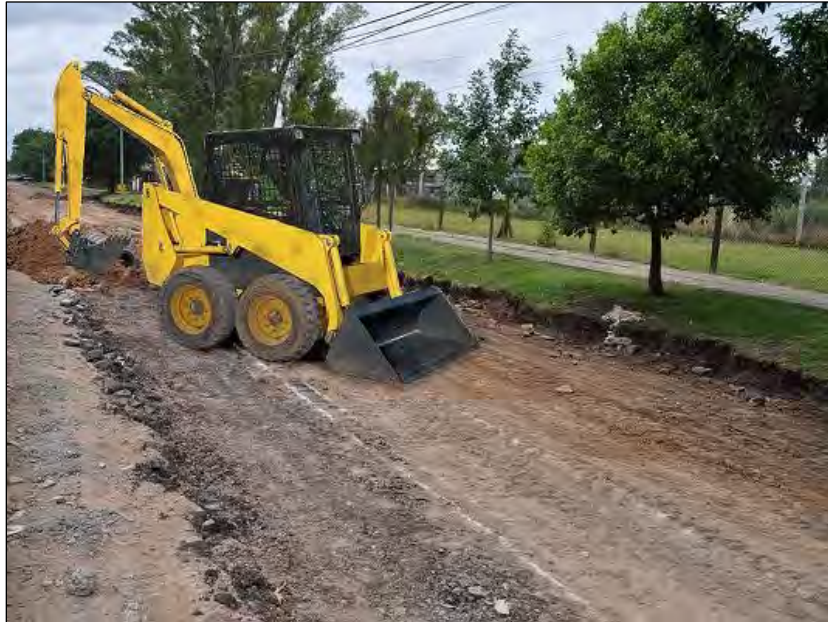
Photo Num. 3.2. Excavation of grading and stripping
