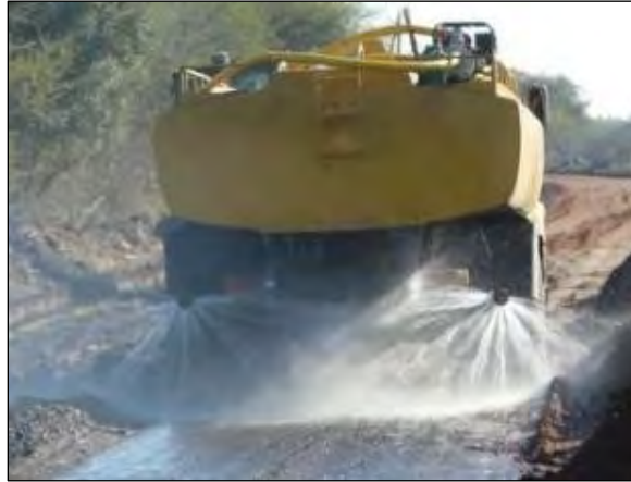
Photo Num. 3.5. Moisture of subgrade material when it is very dry Source: PIO SAS, September 2015.
