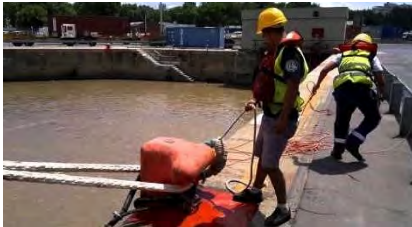
Photo Num. 3.3. Installed bit ton a dock Source: PIO SAS, September 2015.
