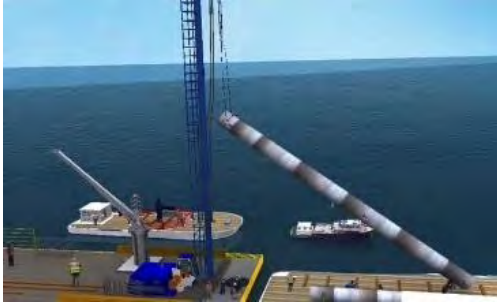
a. Placement of the pile in position to be driven
