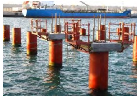
d. Capital or prefabricated ring installed in the pile
