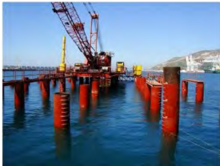
c. Metallic platform and crane installed
