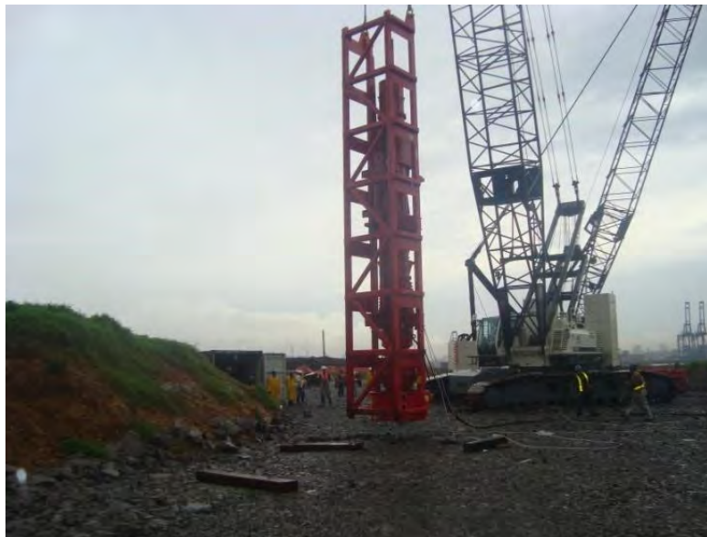
Figure Num. 3.25. DELMAG hammer and crane
